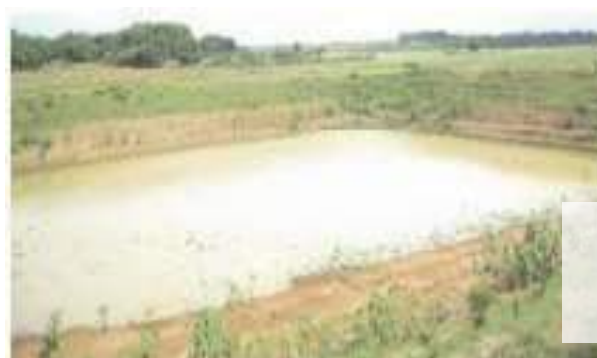
Community Tank Renovation
