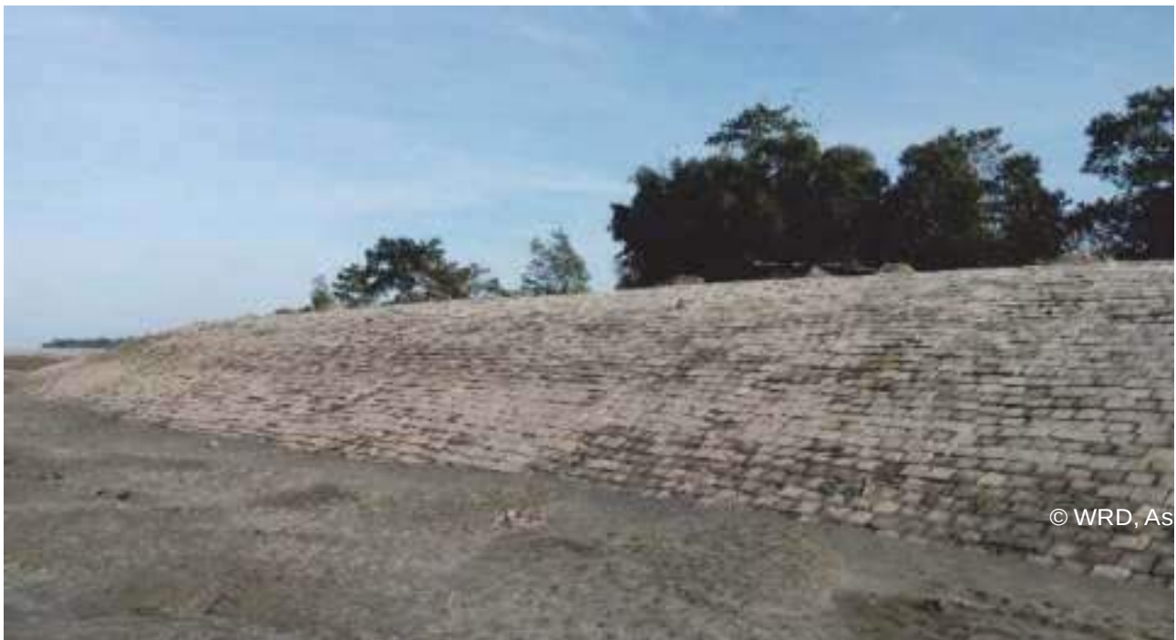
Use of CC block revetment on dyke
