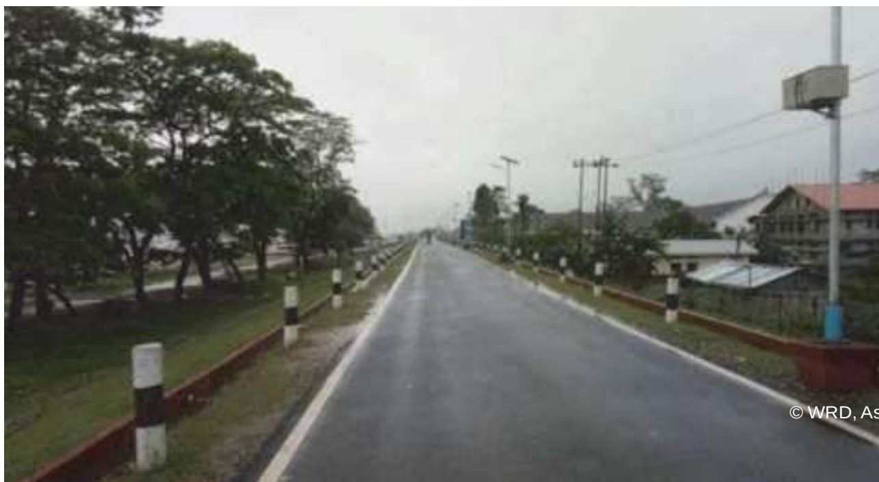
Walking Path built on the Dyke
